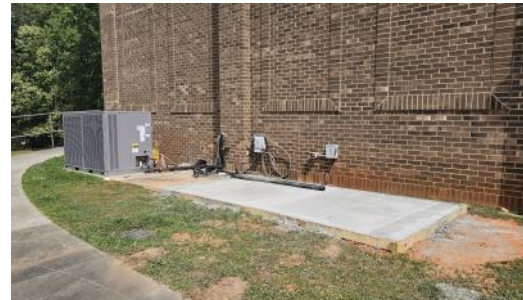
Expanded slab for new units coming .
