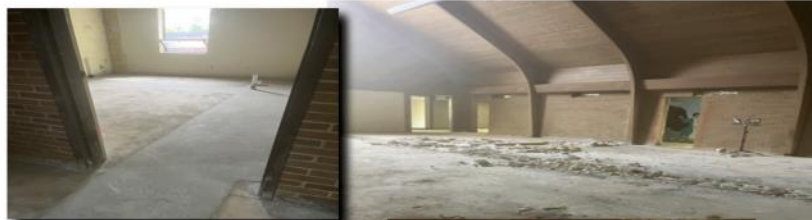
Top right and right: Trenching of sanctuary floor.
